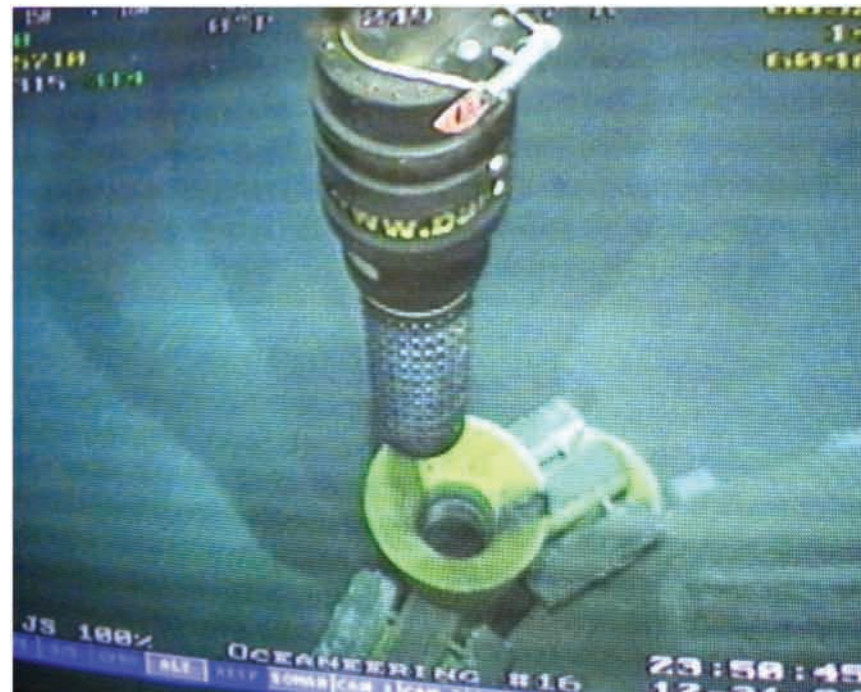
Subsea mooring connection
